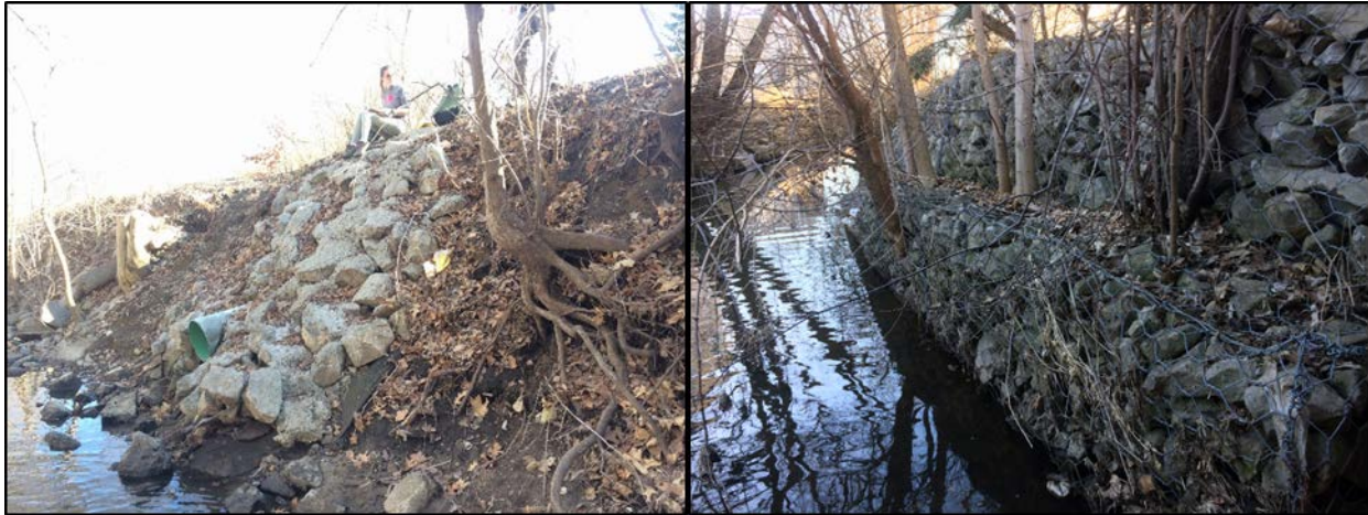
Figure 46. The image on the left shows a poor example of bank stabilization, where debris and cement was slopped into the stream and down the bank. Concrete is not a good way to stabilize it gives no movement for the stream and will speed up the waters movement causing more erosion to occur. The image on the left is between UNI's campus and College Street where apartments are being built, these apartments are right on the streams edge and rip rap was implemented to control bank erosion throughout this area. This kind of stabilization will help to prevent erosion, but not allow the steam to move at all.
