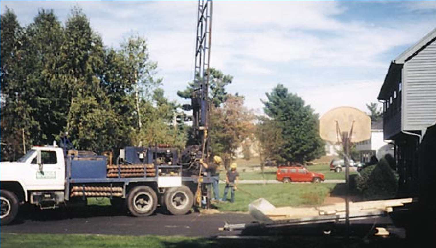
Drilling for the water table
