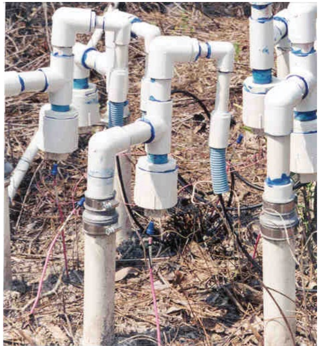
Figure 5.—Proper installation and monitoring of equipment as described in the Hydric Soil Technical Standard is required to collect data regarding proposed additions, deletions, or other changes to the hydric soil indicators.
