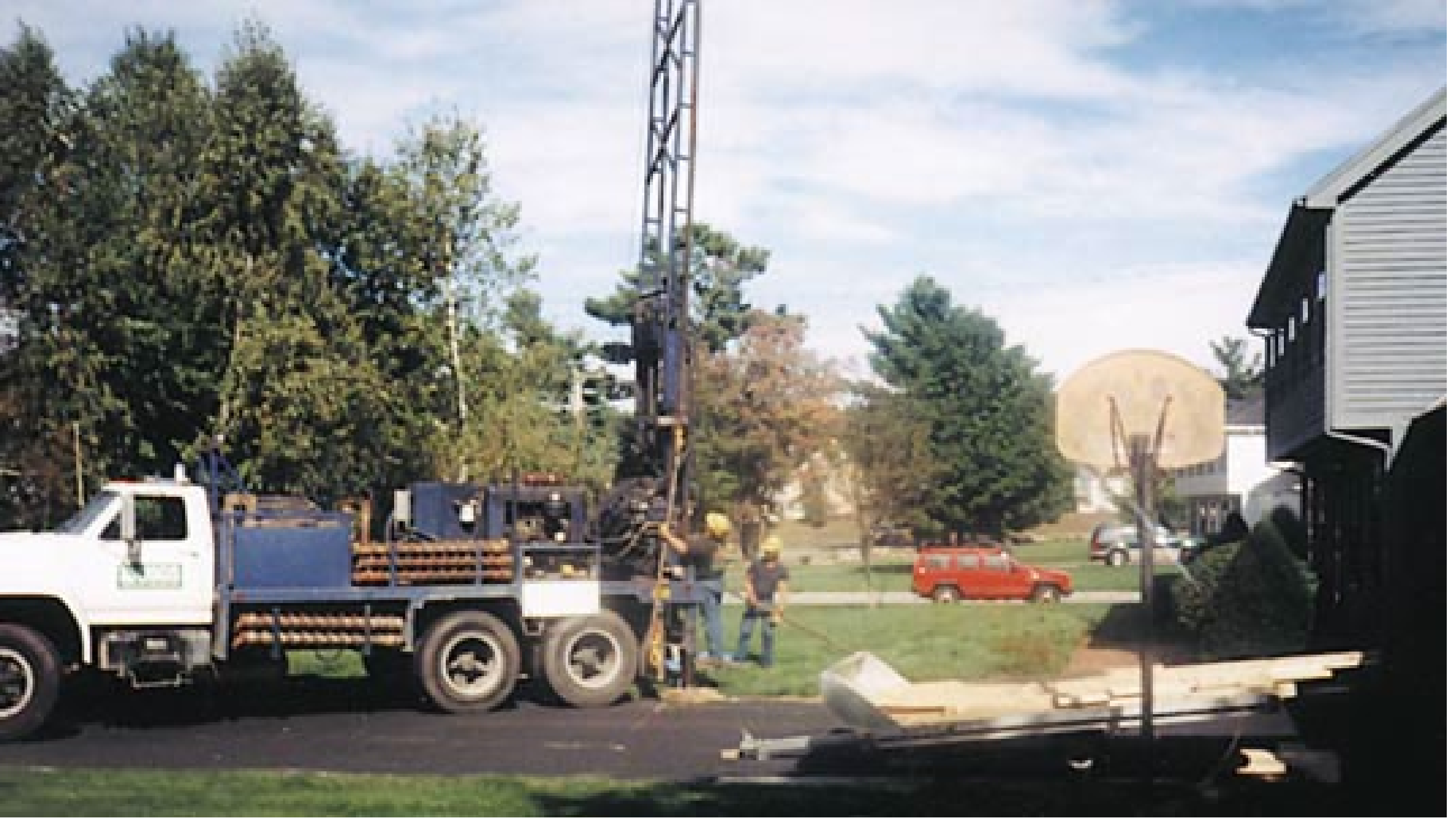
Drilling for the water table
