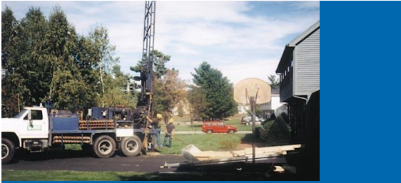
Drilling for the water table
